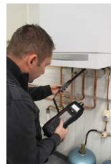
Ambient CO checking
