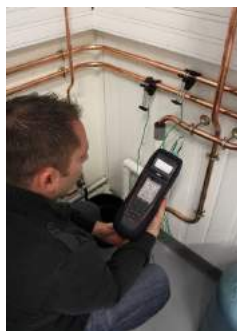
DHW network temperature
