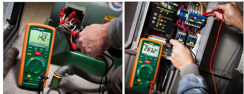
Checking voltage on a lathe and insulation test on pump motor
